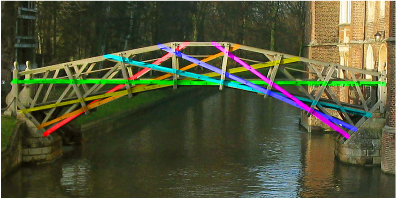
Flickr - Duncan Hull (image highlighting tangential members of the bridge)
